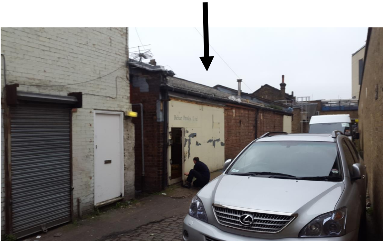
Image 1: The existing building from St Albans Place
