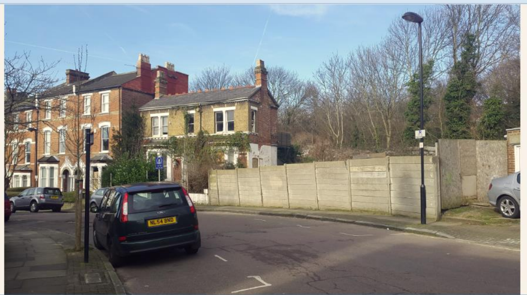
Image 1: The existing building from Blythwood Road
