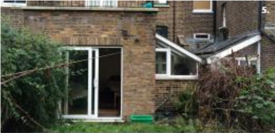
Image 1 - View of rear elevation and part of rear garden
